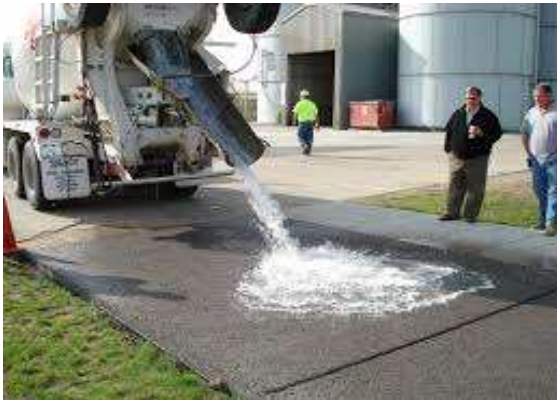
Fig 2. Pervious concrete pavement
