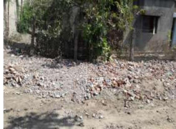
Fig. No. 5 Area selected for the parking (Before completion of work)
