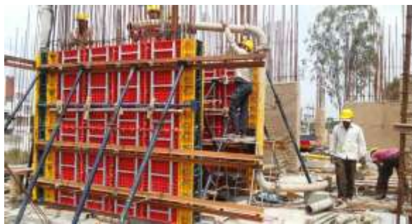
Fig.2 NOVA PLASTIC FORMWORK
