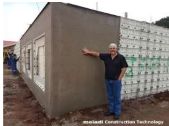
Fig.3 MOLADI PLASTIC FORMWORK
