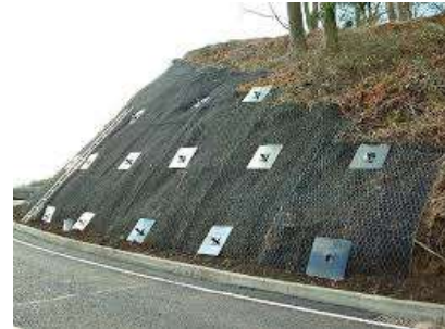
Fig. 1: Soil Nailing
