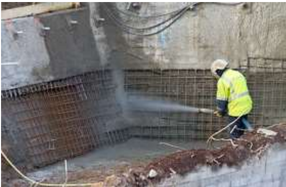
Fig.7: Shotcreting process with compressor
