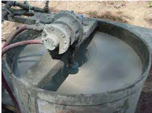
Fig.4: Grout Mix and Mixer
