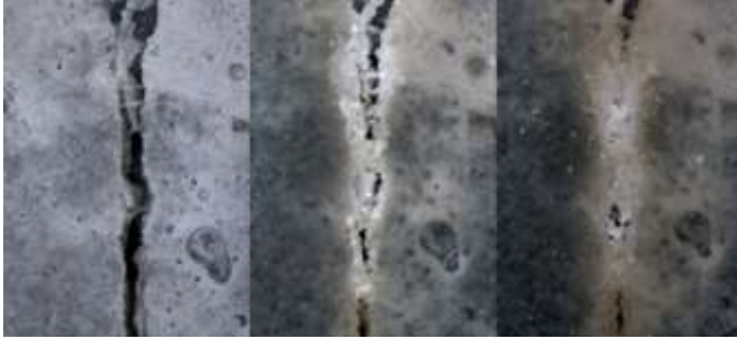
Figure 5: Stages of healing the concrete
