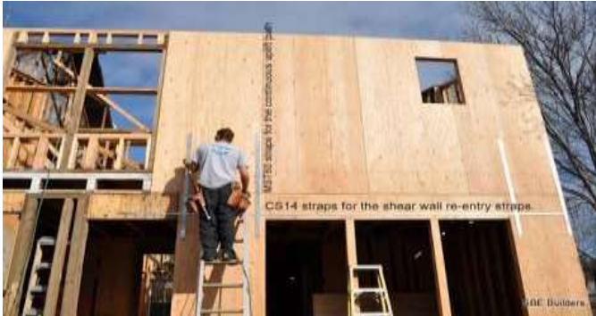
Fig. 2: Plywood Shear Wall
