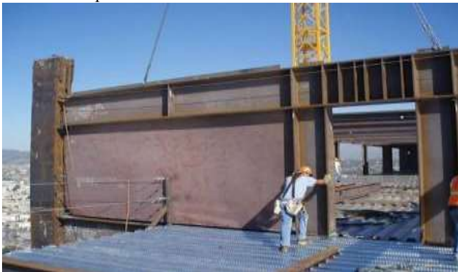
Fig. 3: Steel Plate Shear Wall
