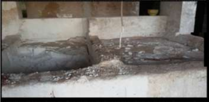
Fig-2.1: Cooling of lime before use in construction
