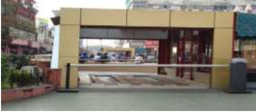
Fig. 2.0 Car Parking System in Kolkata
