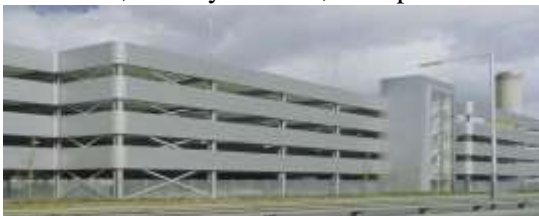
Fig 1.0 The Genesis multi-storey car park, World Cargo Centre, Heathrow
