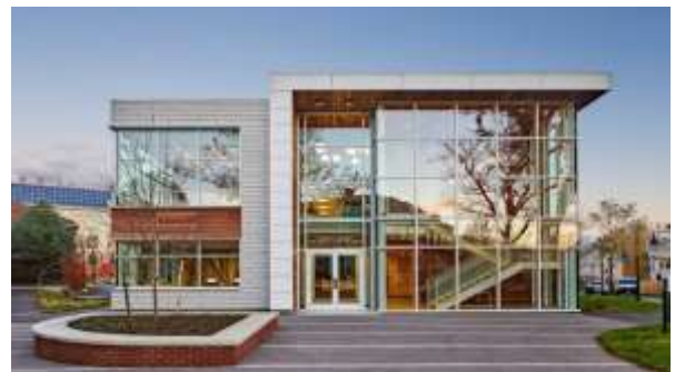
Fig.1. Building Integrated With Photovoltaic Glasses
