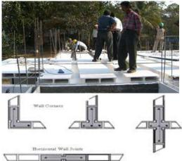
Wall to wall 'L', 'T', '+' angle joints and horizontal wall joints are made by cutting of inner or outer flanges or web appropriately and infill of concrete with vertical reinforcement with stirrups for anchorage. Various construction joints are as follows.
