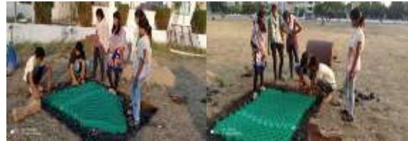
Fig. Spreading of geocell
