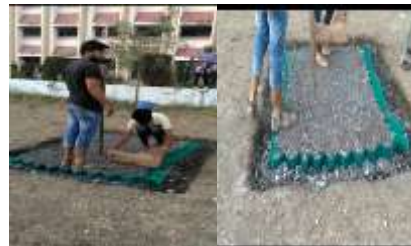
Fig. Compaction of filler.
