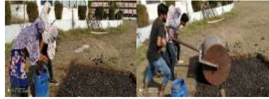
Fig. Roller compaction
