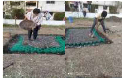
Fig. Filling by material
